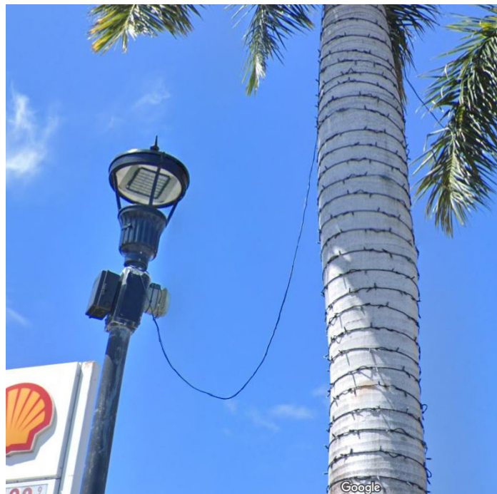
UNSAFE WIRING
